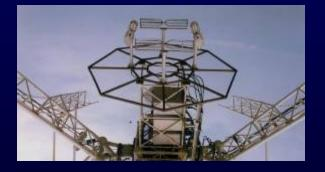
Antenna primary feeds are placed on **a rotating turret** near the focus of the dish
