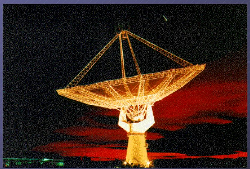
Note the light, see-through structure reducing wind forces, weight, and cost
