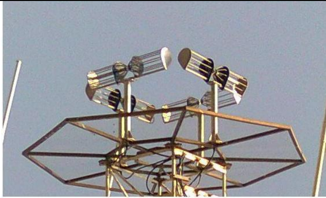
Fig b: 150MHz Folded Dipole
