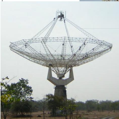
Painting: Very important for maintaining the health of the mechanical structure Takes  $\sim$ 3 months to paint one GMRT dish !
