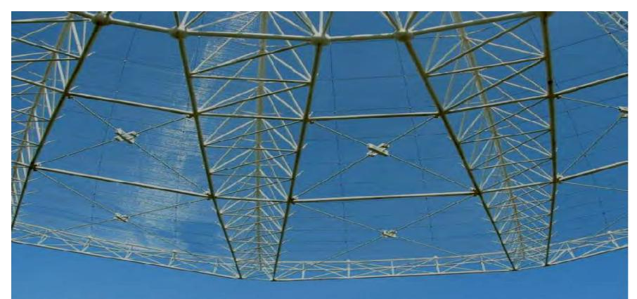
•7% solidity with 0.55 mm diameter Stainless Steel (SS) wires spot-welded at junction point to form a surface with 10x10 / 15x15 / 20x20 mm wire-grid.
