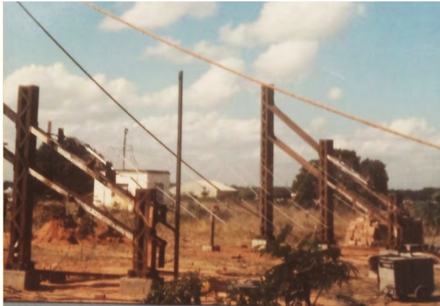
Initial photo the development of rope truss with mesh attached.
