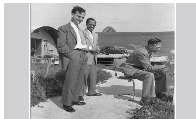
Fig 3. Stanford March 1958. Joe Pawsey puts his carved signature on pier East 1 of the Stanford Microwave Radioheliograph under construction. From the left Ron Bracewell, Govind Swarup and Pawsey. This pier is now part of the Bracewell Radio Suidial at the Very Large Array in New Mexico (Noon pier). Swarup's signature is on pier East-2 (10 am pier)
