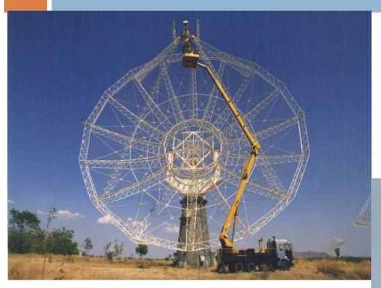
High Lift Platform for servicing front-end amplifiers, electronics and structural maintenance
