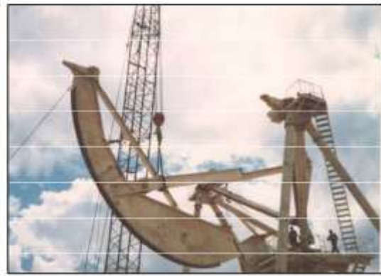
xi. Installation of EL bull gear mount and connection with EL Plummer mounts
