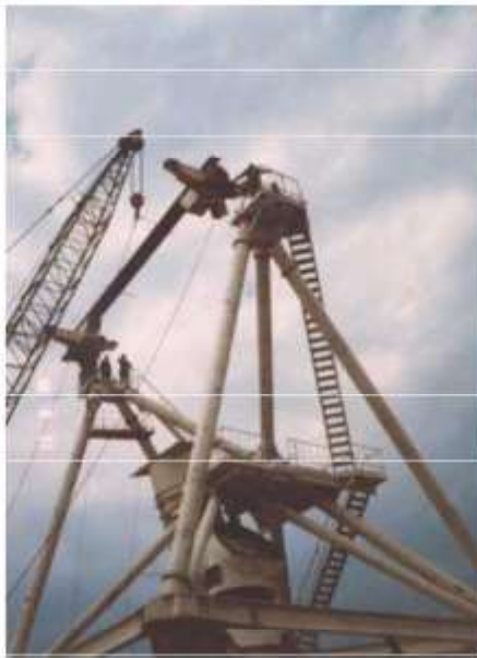
xi. Installation of EL bull gear mount and connection with EL Plummer mounts
