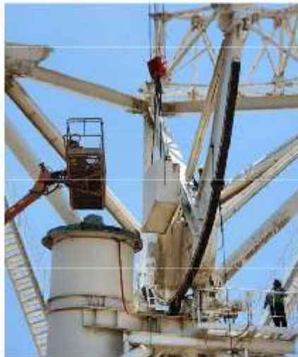
xii. Installation of Counter weight
