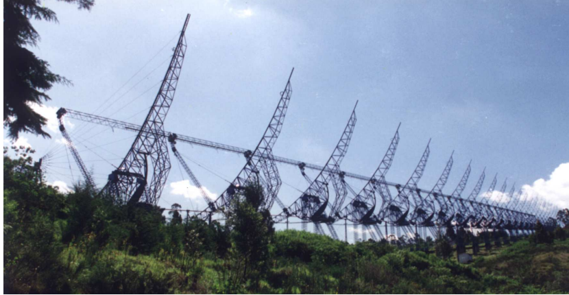
Figure 5. The Ooty Radio Telescope is a cylindrical paraboloid of reflecting surface, 530 m long and 30 m wide, placed on a hill whose slope is about 11 degree (in the north-south direction), which is the same as the latitude of the location.
